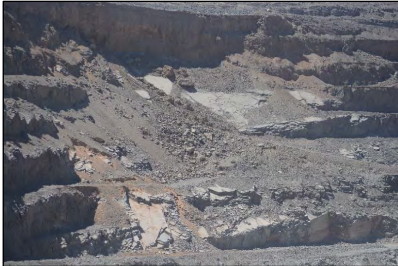
Figure 2: Planar failures on the Jwaneng mine eastern slopes mined with conventional vertical batters
